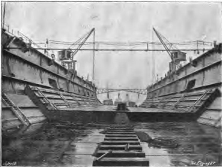
Fig. 513.—Centre Pontoon Floating Free. Rest of Dock being Sunk.
